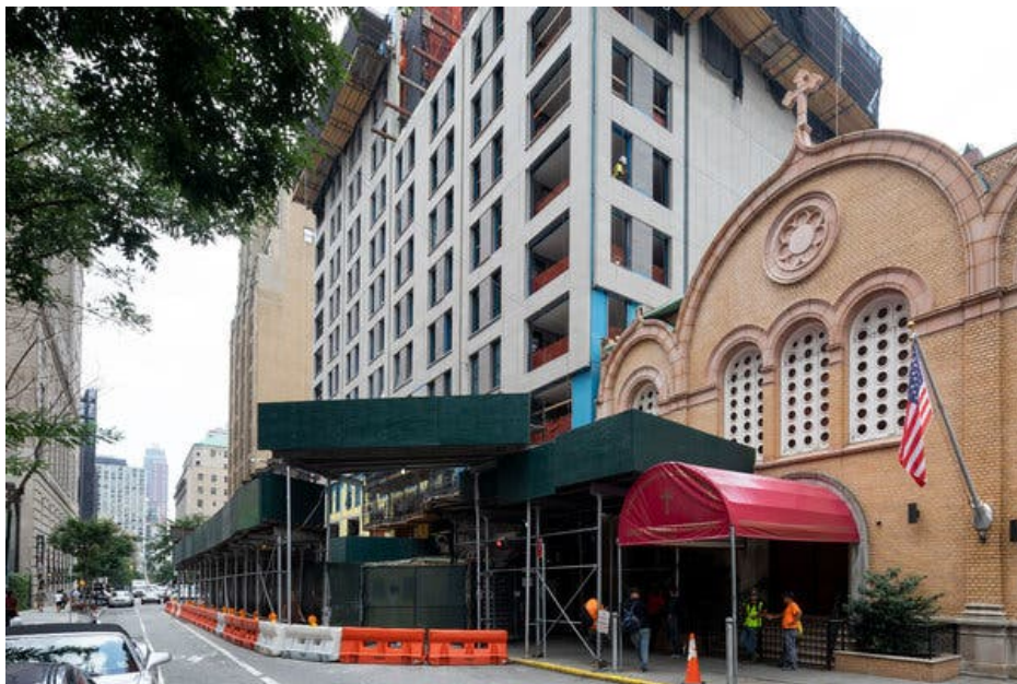
The Symon, a 59-unit condo under construction at 76 Schermerhorn Street in downtown Brooklyn has a private nine-car automated garage. Credit Katherine Marks for The New York Times
